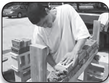
Trainee learns bricklaying skills on the job site
